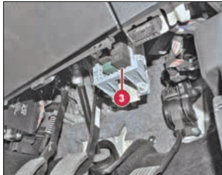
Fuse location- Cabin compartment
